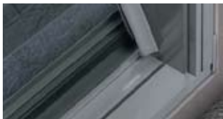
The seals at the corner joints are hidden.
